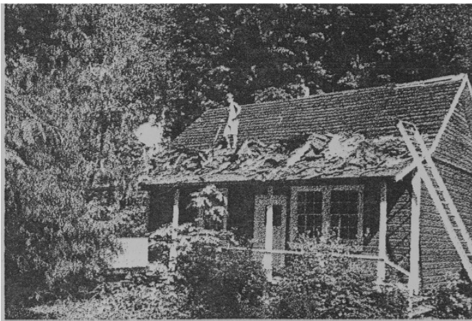
1989 removal of the old roofing material
