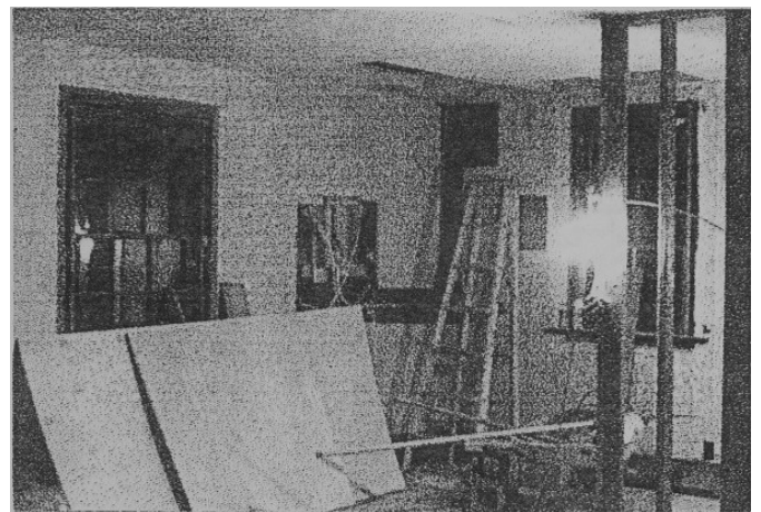
1982 Interior view of the schoolhouse during renovations
